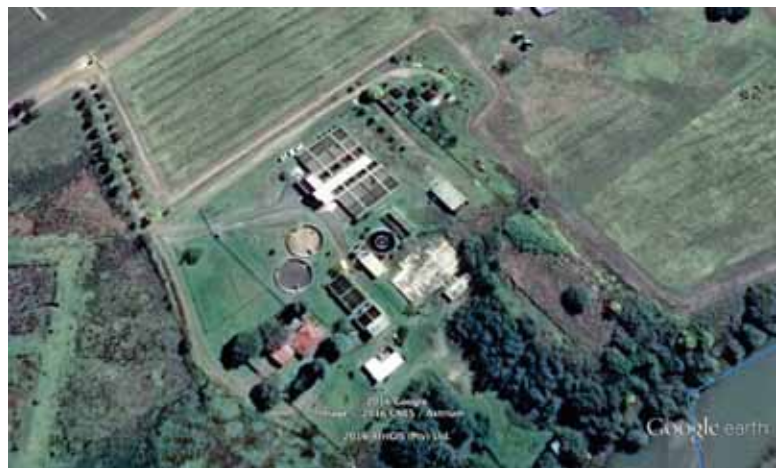
Standerton Water Treatment Works
